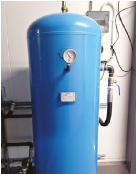
Nitrogen generating system holding tank. It can be used in cold rooms or a mixing box to lower oxygen levels for fumigation.
